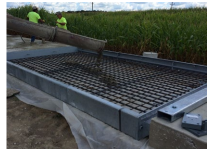
VTC19X Rebar and Concrete
